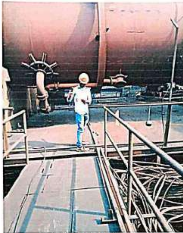
DRI 2 KILN AREA
