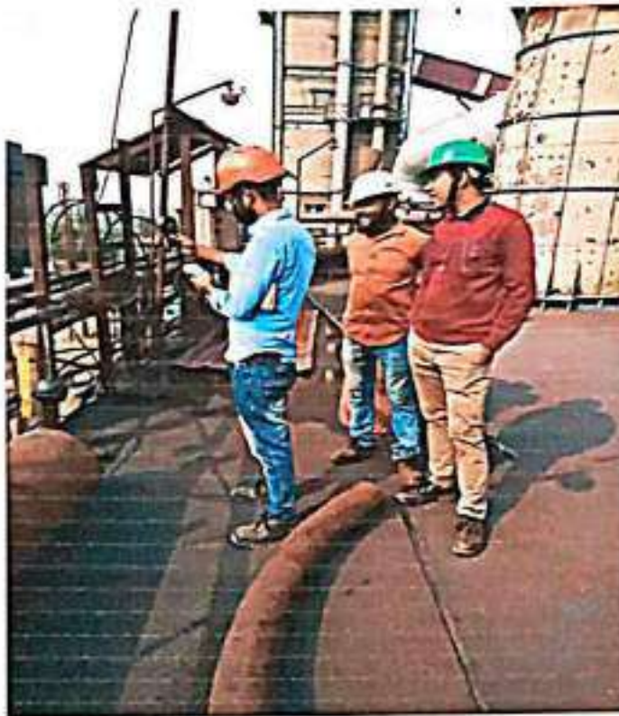
Pellet 1 Cooler Floor Photo
