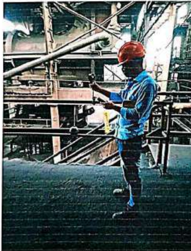
DRI 3 DSC AREA
